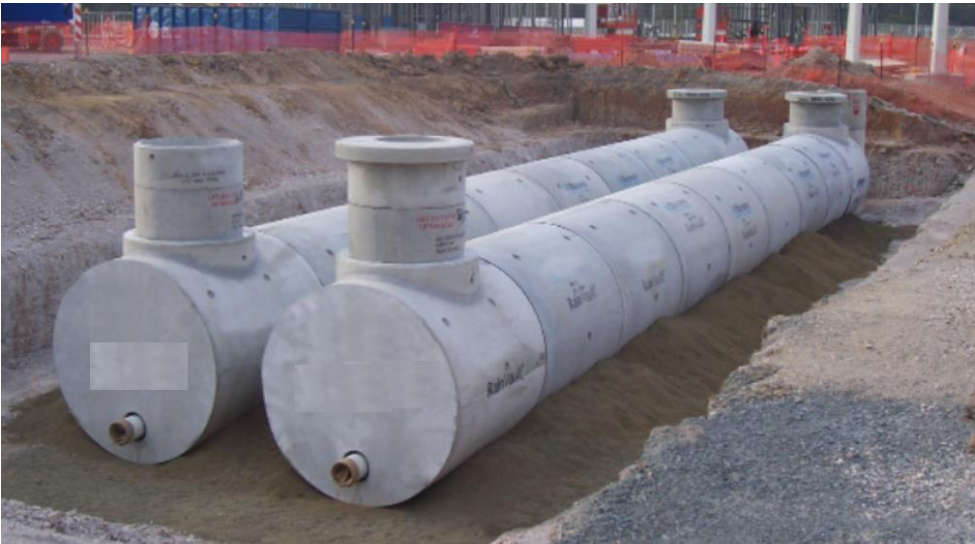
Figure 9 - Below ground rainwater tank
